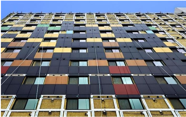
Figure 4. Retrofitting of residential buildings in Canada using solar photovoltaic (PV) modules..
