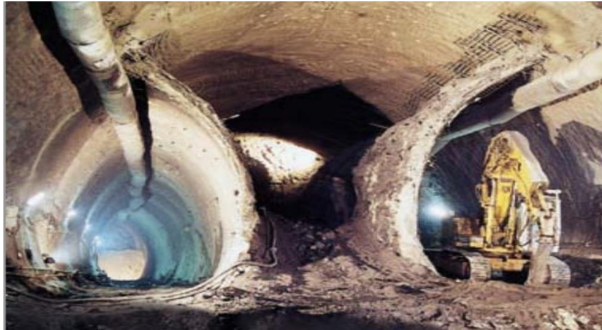
1- picture. Underground Structure Excavation
