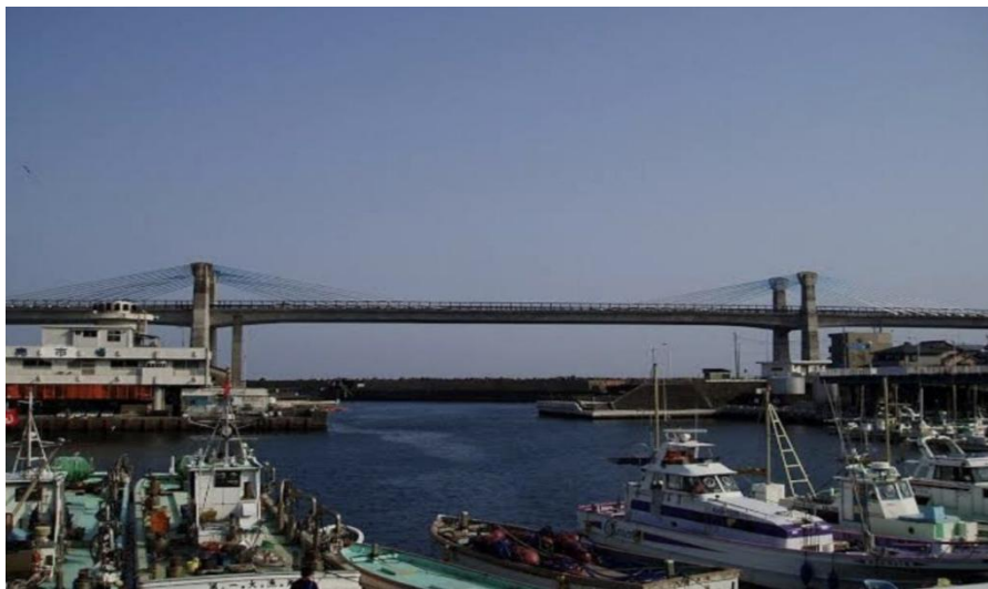
2- picture. “Odawara Blueway” bridge
